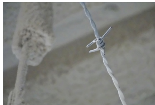
Fine dust deposit (in the background)
